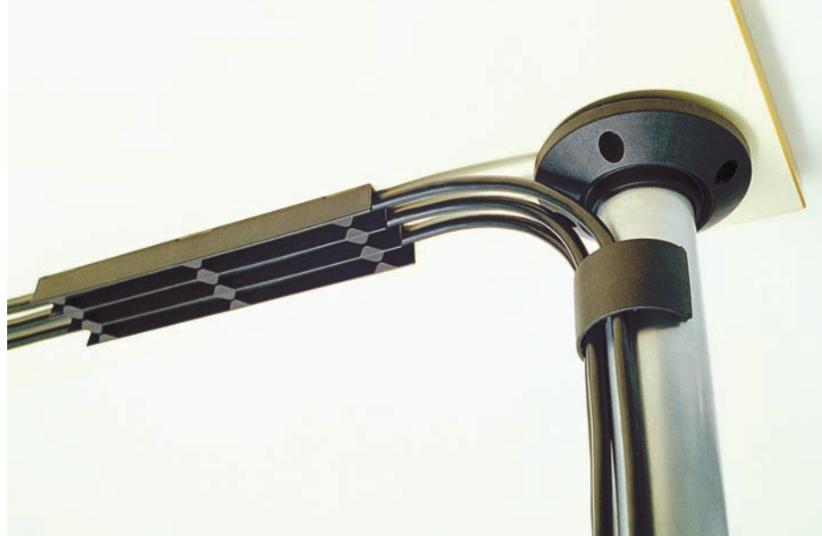
Cables housed in cable track, secured to leg with cable clip
